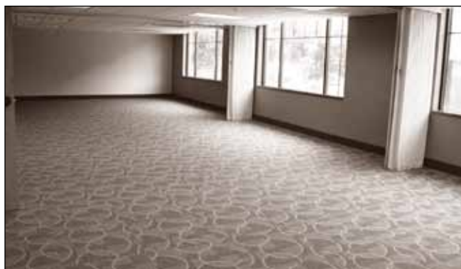
Education rooms were remodeled into more flexible space, plus the old glass block was replaced with larger, energy-efficient glass panes overlooking a courtyard.
